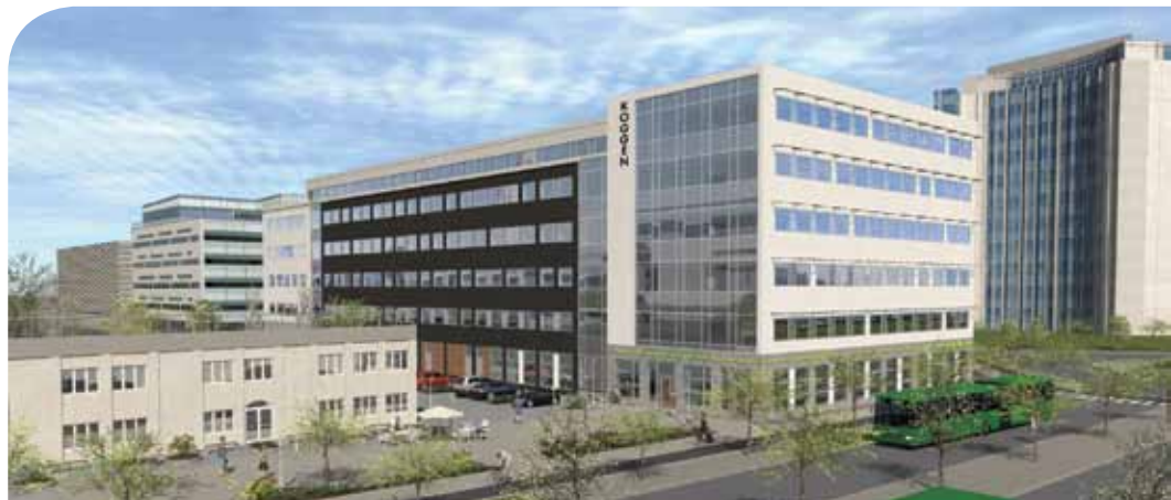
Koggen 2, Västra Hamnen in Malmö: The first BREEAM Excellent building in Scandinavia
